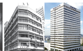
The initial stages of the Construction Building (L) Jun. 1986 Completion of the Construction Building
